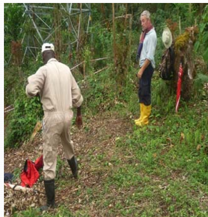
Preparation for clearance around power lines.
